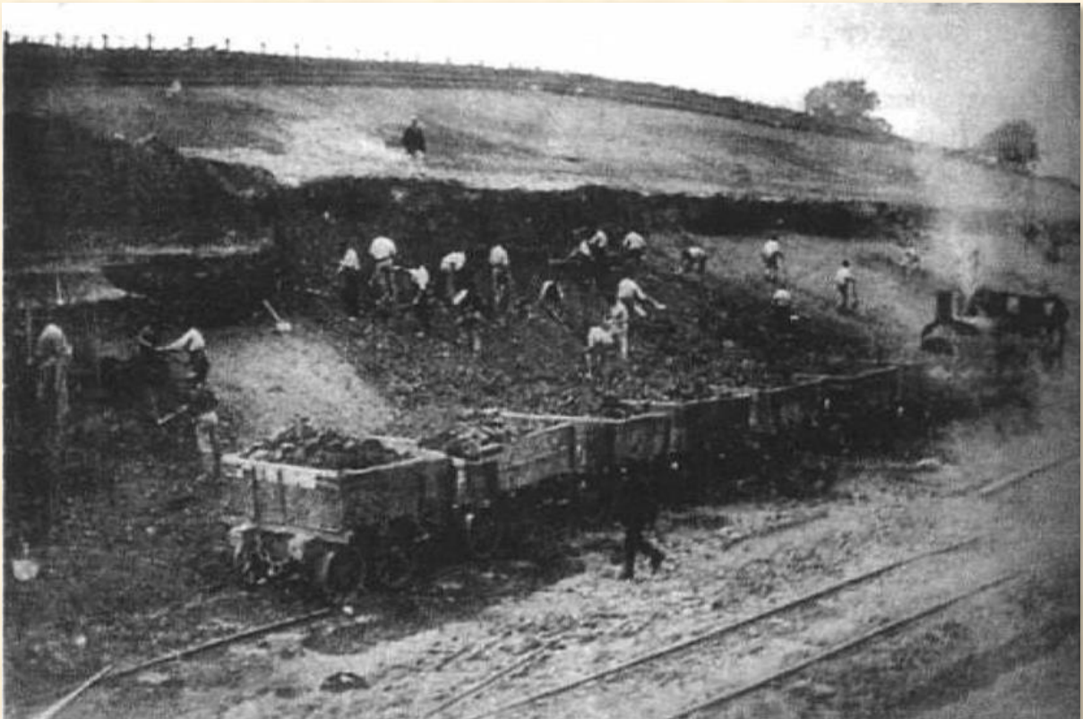
Railway labourers or 'navvies' digging a cutting in 1872 on the Worthington section of the new branch line from Derby. They also used a mechanical excavator known as a 'steam navvy'. This single-track extension from Melbourne reached Ashby-de-la-Zouch in 1874. James Haywood probably knew the labourers in this photograph, and may be among them. (Hand-Me-Down Hearsays, Simon Jones and Jamie Wigmore, 2003 – Breedon on the Hill Parish Council )
