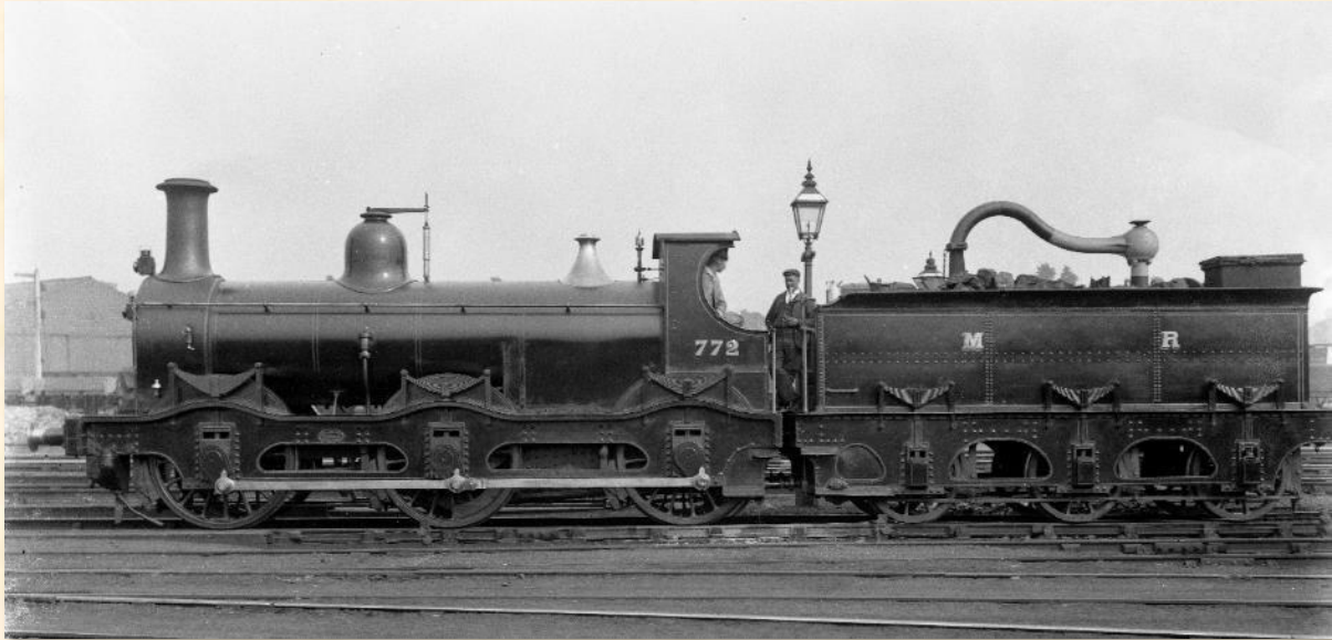
A driver and fireman in the cab of a Kirtley Class 700, built between 1869 and 1874. It is seen here before 1907 when the Midland's numbering system was changed. As a fireman in the 1870s, and as a driver from 1889, Thomas would have been familiar with these locomotives. (Mick Hymans Collection, with thanks to Charlie Verrall )
