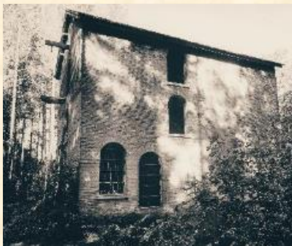
The 'Seldom Seen' engine house of Plumbley Colliery, nine miles (14.5 km) north-west of Elmton. A PC Clifford, possibly George rather than Thomas, arrested a tramp here on 23 August 1884. (With thanks to Spike on Flickr )
