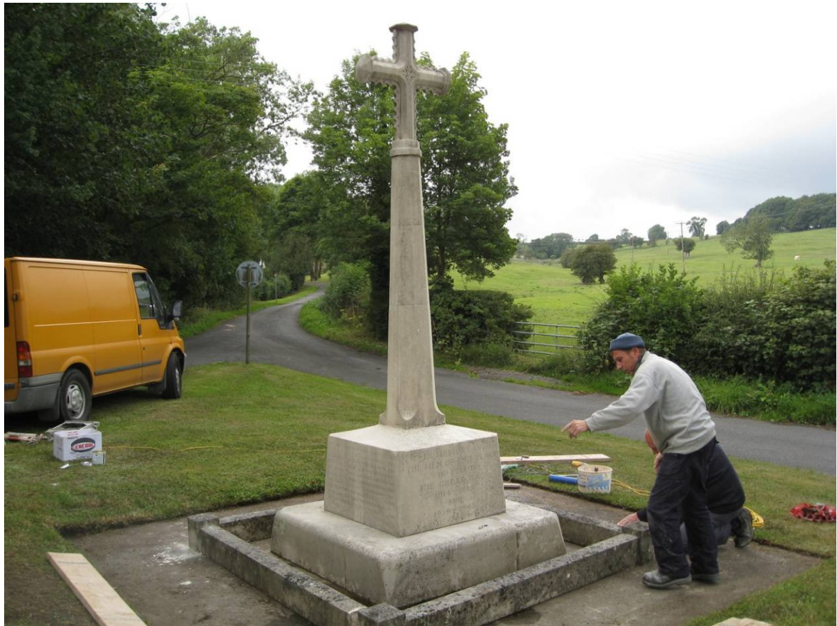
Workmen in August 2010 cleaning and repairing the war memorial.
